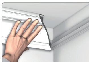
Attach the cornice to the rail and against the ceiling
